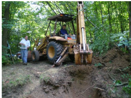
The east bank required backhoe work.
