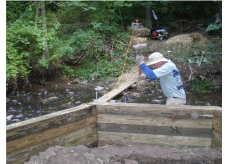
Chauncy driving home the nails in the foundation wall.
