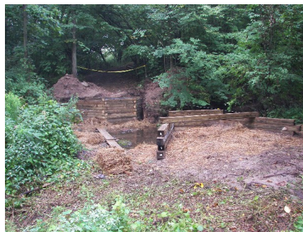
Reading for the decking.
