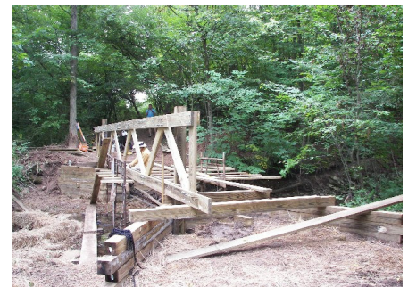
Starting to look like a bridge.
